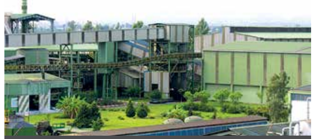
Kromsan Chromium Compounds Plant - Mersin Turkey
