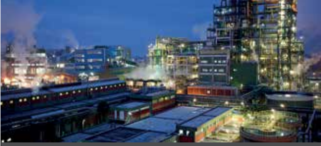
Soda Plant - Mersin Turkey
